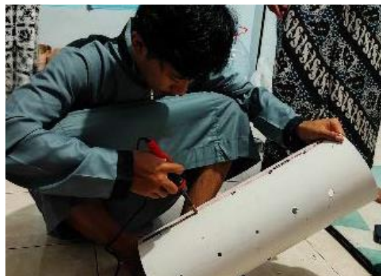
Figure 6. Biopore Construction
